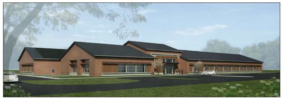
Photo courtesy of Chatham County Schools
